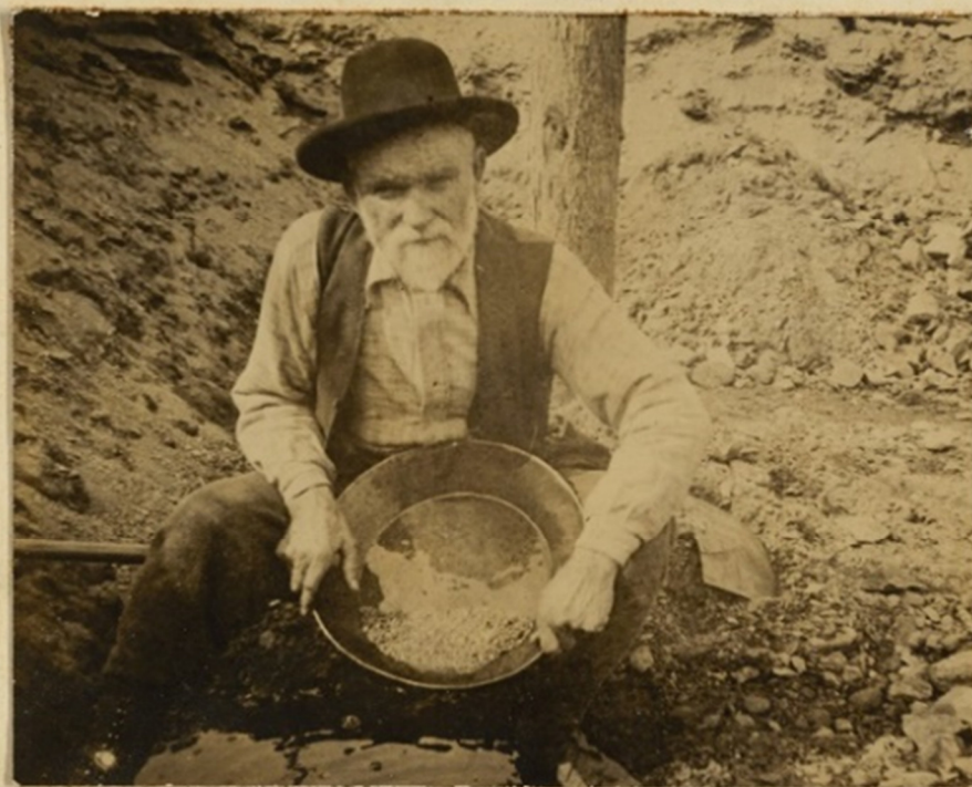
JOE IRVING, FORMER, ON CLAIM OF DICK LOWE, WITH HIS PAN OF GOLD WORK TAKEN FROM ONE PAN OF DIRT, (ABOUT 25 SHOVELS TO A PAN).
